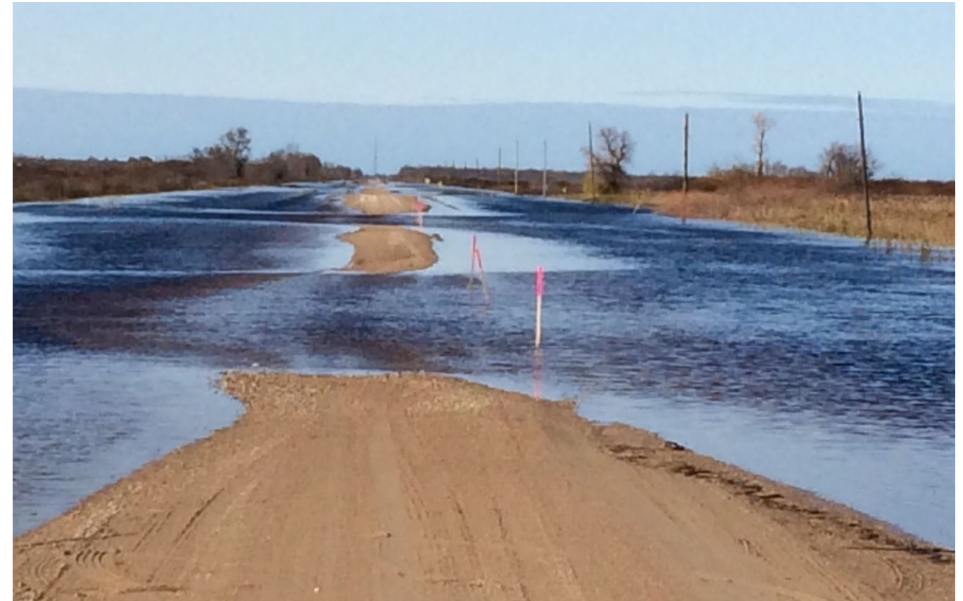
Roseau River overflowing Roseau County Road #7, fall 2019
